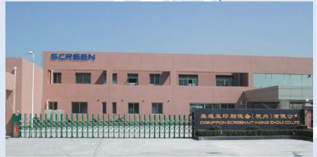
MTMC office building
